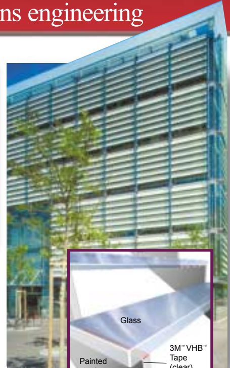
Glass steps bonded to varnished steel frame, Tamedia Building, Zurich, Switzerland
