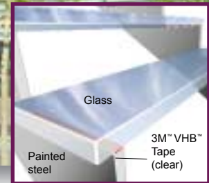
Glass steps bonded to varnished steel frame, Tamedia Building, Zurich, Switzerland
